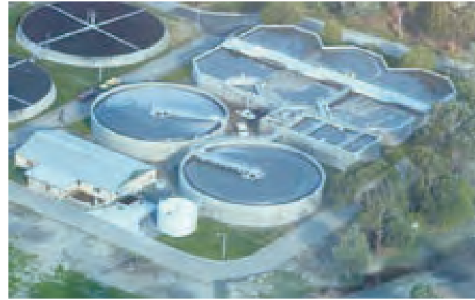
Figure 10.7 An aerial view of a sewage plant
